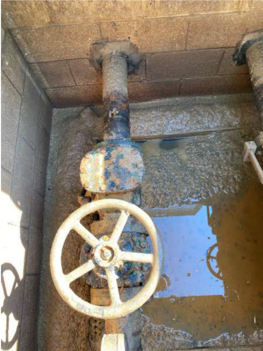
Photo 5 Valve Vault No. 3 – Interior with crushed stone bottom
