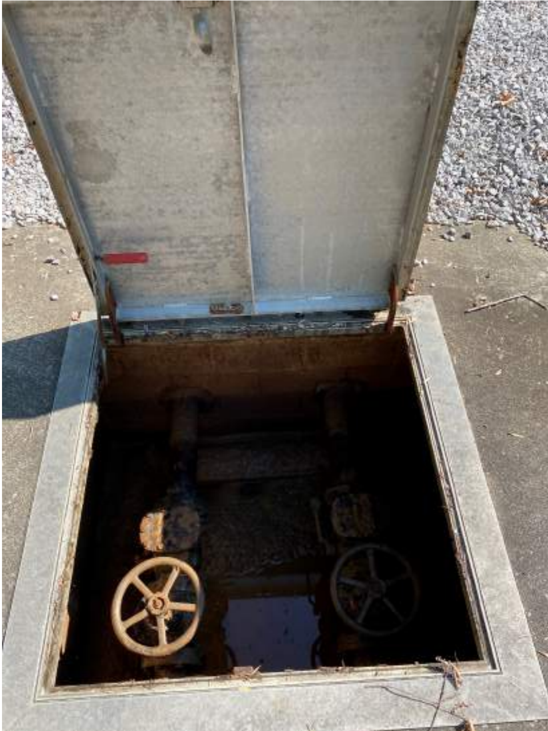
Photo 3 Valve Vault No. 1
