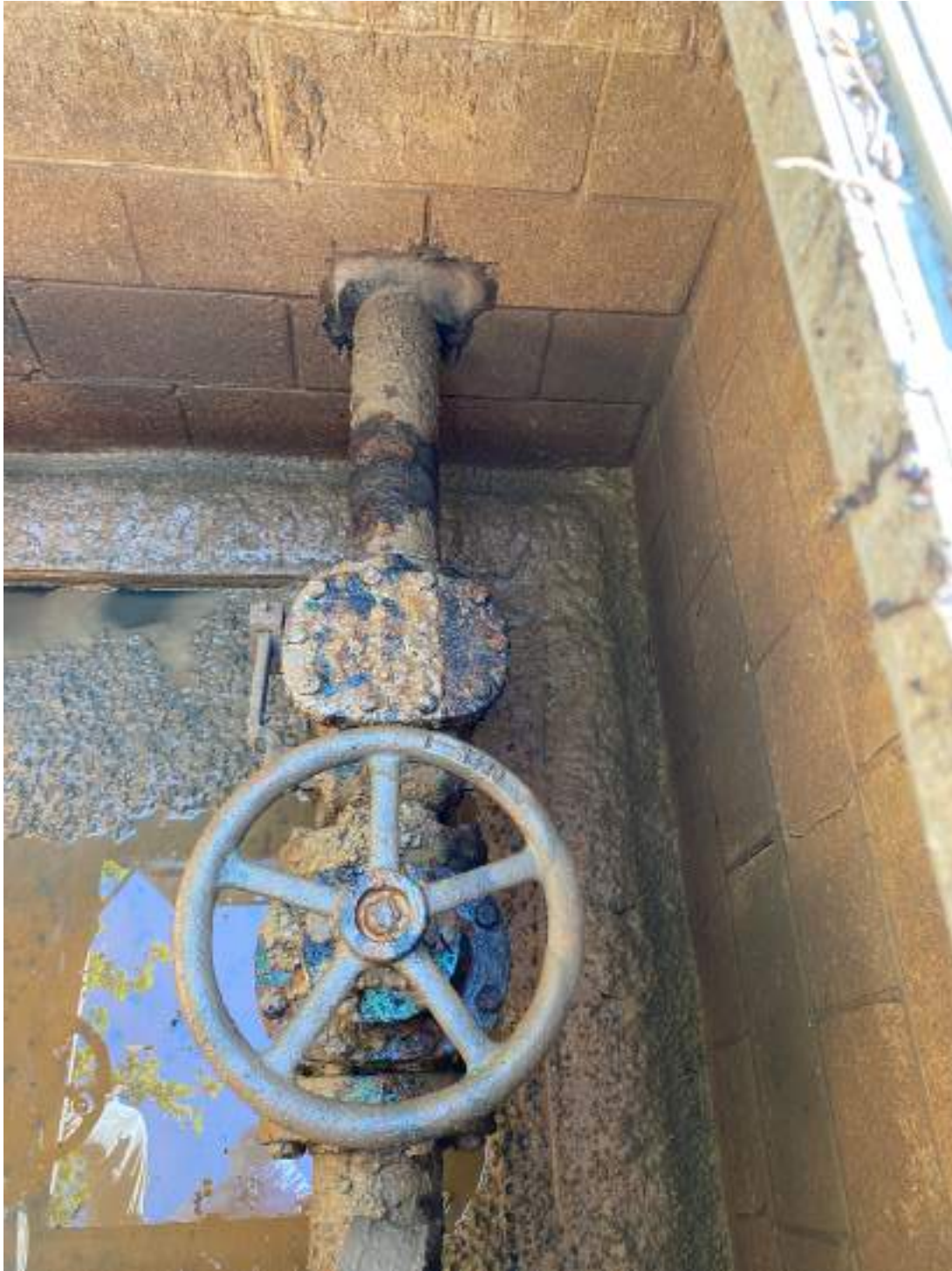
Photo 4 Valve Vault No. 2 – Interior with crushed stone bottom
