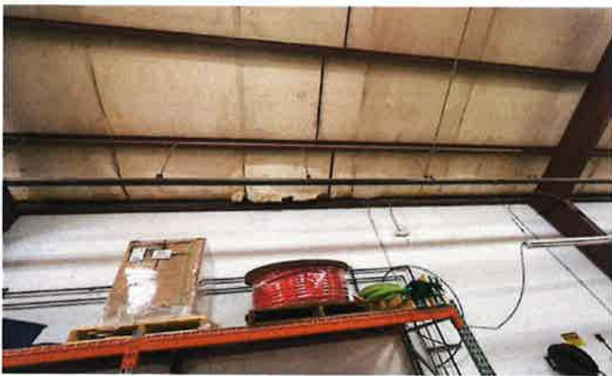
Sewer Complex Garage Roof Leaks
