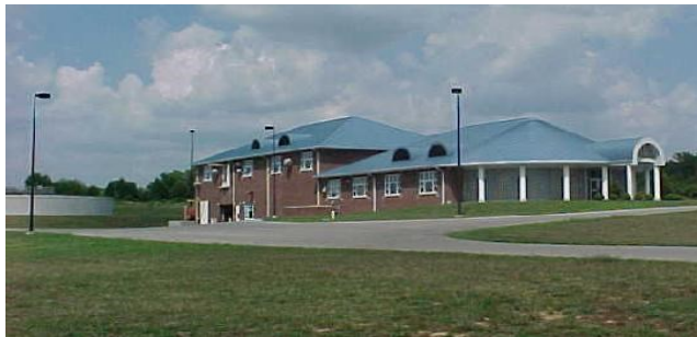
HWEA's Moss Water Treatment Plant
